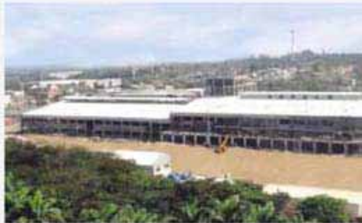
Construction of new culinary plant at Nanjangud
